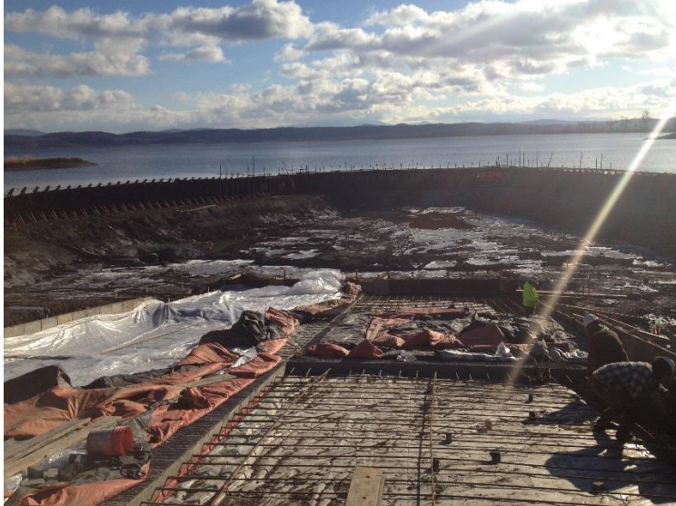
Facing east, looking at a port-a-dam used to dewater Lake Champlain in order to dredge the lake bottom and install the double land boat ramp.
