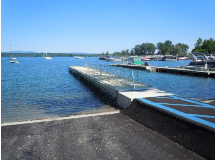
Similar view as the above photo after the port-a-dam had been removed and the ramp installed along with the 70 ft ADA accessible dock and walkway.
