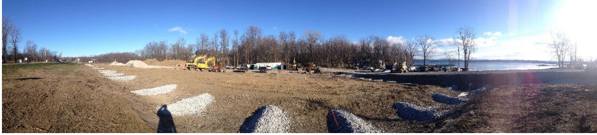
Figure 1. Panoramic view of the active construction of the John Guilmette Fishing Access Area parking lot. December 2014 looking north from US Rt 2 in Milton.
