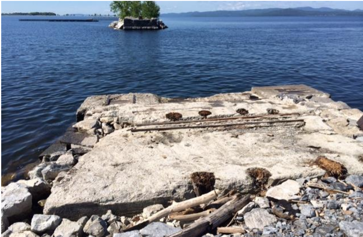
Figure 3. Before and after photos looking south, towards the Colchester causeway, at the of the Allen Point Fishing Access Area fishing platform, South Hero.
